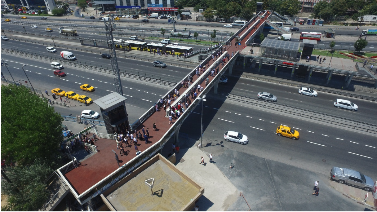
Figure 2. The view of Cevizlibağ Metrobüs Overpass.
