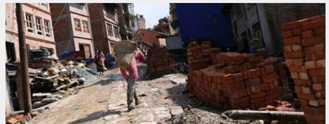
95% of buildings damaged in Khokana, Kathmandu in the 2015 Gorkha earthquake. Credit: Tomorrow's Cities Project
